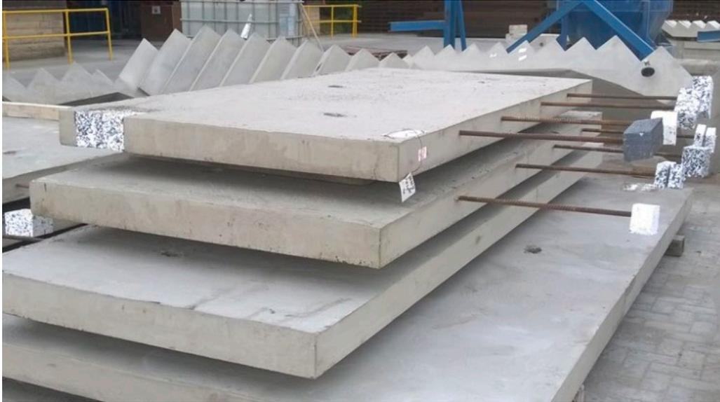
Figure 4 – Simple RC slab with cast in bars for tying back to the main floor slab.
