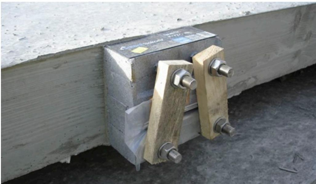
Figure 2 – Close up of cast in thermal breaks.
